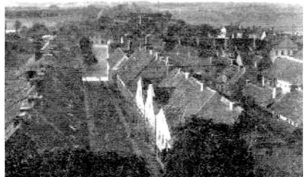
1. The damages of the First World War in a German little Town; Gerduan before (1915) and after (1926) the restoration (Düwel 2001, P. 64)
