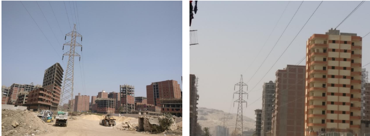
Fig. (9.34) High voltage towers passing through the residential buildings in “El-Moalimeen/El-Arbieen/El-Sadat” area
