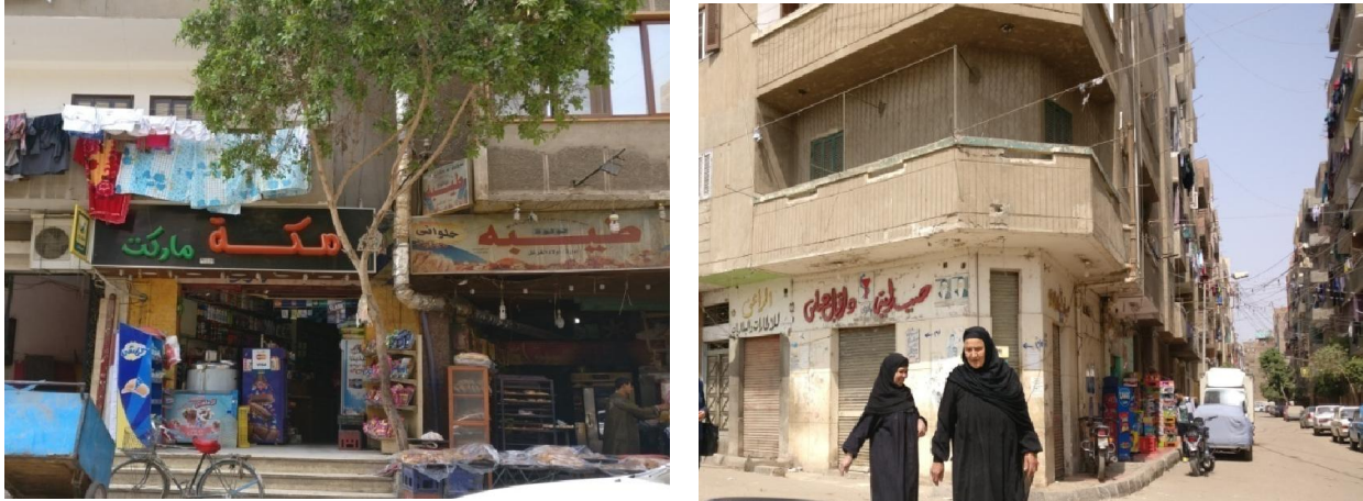
Fig. (9.28) Examples for the usage of the gourd floor of the residential buildings for commercial purposes in “El-Moalimeen/El-Arbieen/El-Sadat” area
