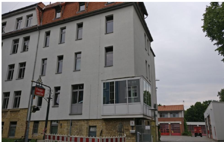
Fig. (9.16) The fire station “Schlauchturm BF Osnabrück”
