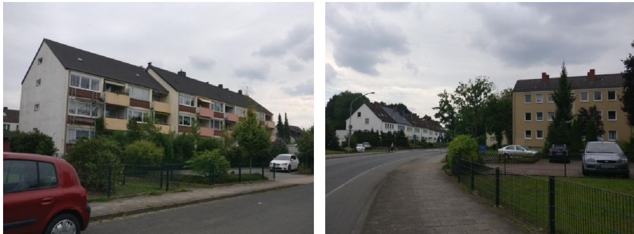
Fig. (9.5) Examples for houses for more than one family in “Sonnenhügel” district
