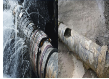
Figure 1.4: The effect of the surge (pipe breakage) published after permission of the owner [59].
