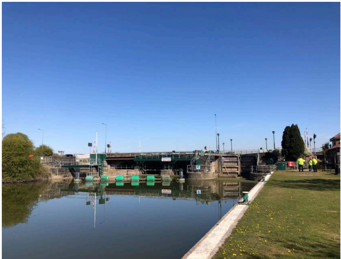
Photo 4 (top) and 5 (bottom): Overlooking the Humber Estuary from Sluice Road and completed construction of the South Ferriby Scheme. Source: Author's archive: April 2021
