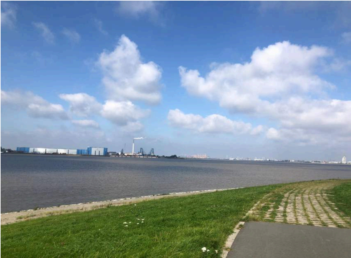
Photo 12: Completed Flood defence scheme along the River Weser. Source: Author's archive: September 2021
