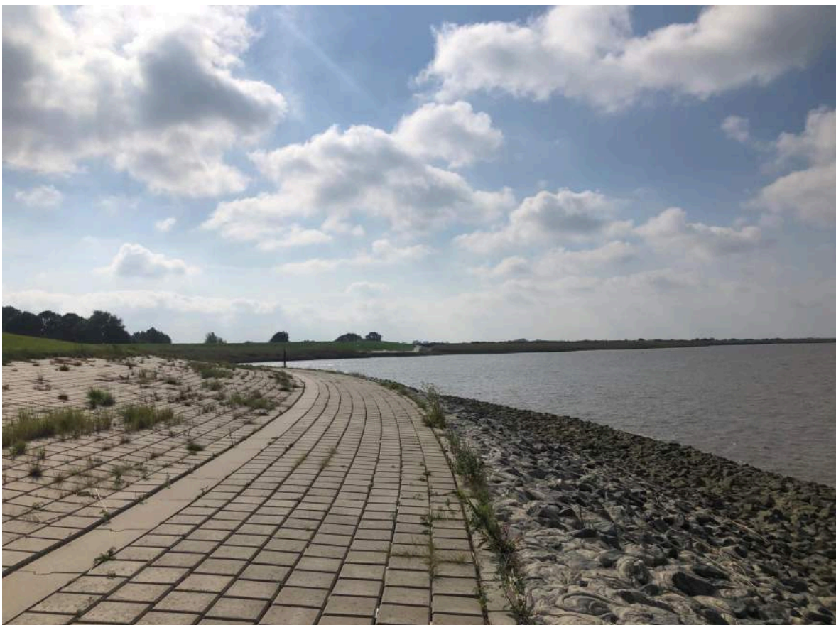
Photo 8: Completed Flood defence scheme along the River Weser. Source: Author's archive: September 2021
