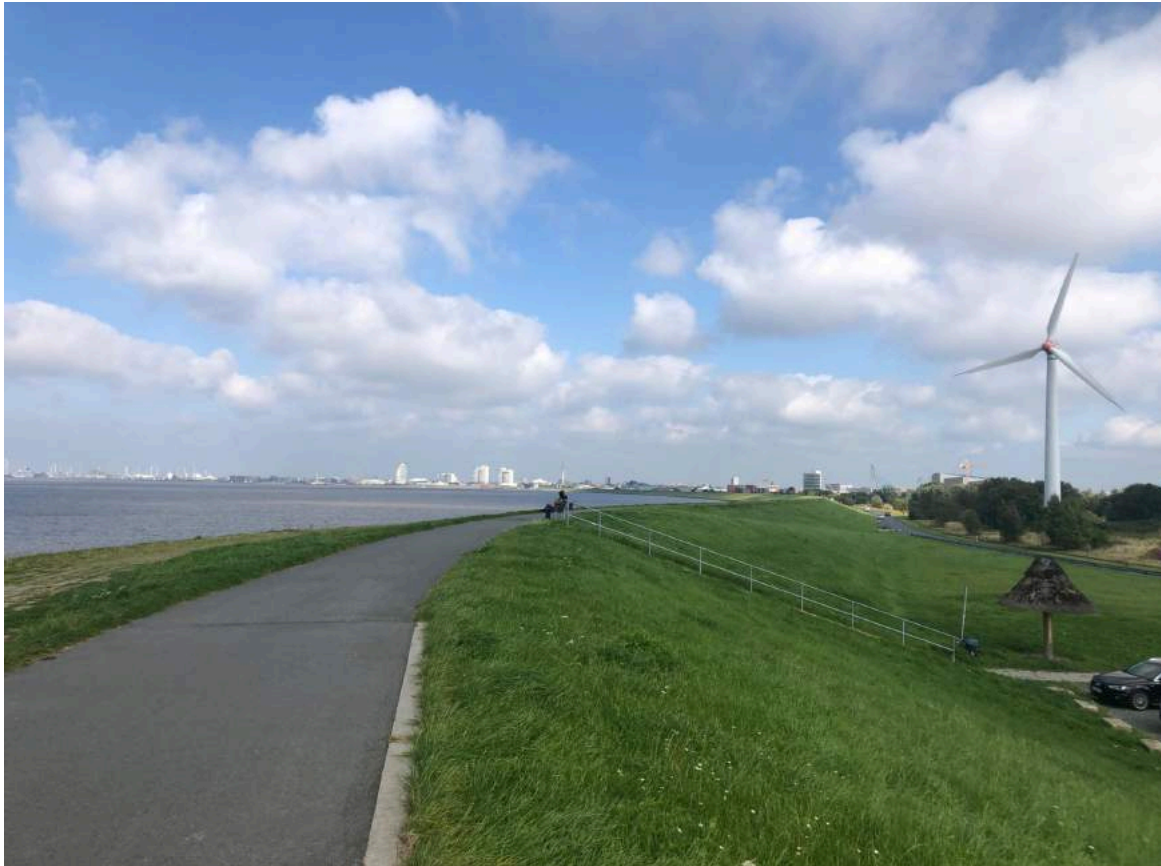
Photo 9: Completed Flood defence scheme along the River Weser with pedestrian path and access for emergency vehicles. Source: Author's archive: September 2021
