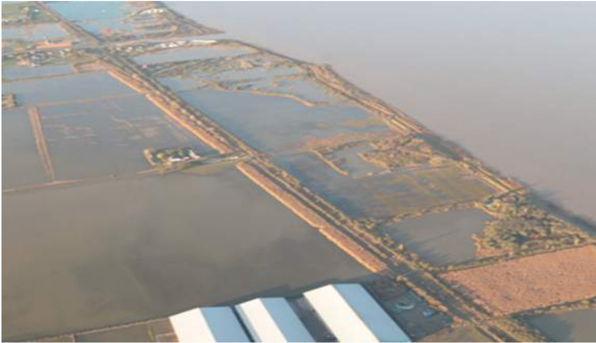
Figure 17: Aerial view after the North Sea flood in 2013 in North East Lincolnshire: Barton, Barrow Haven, and New Holland. Source: Environment Agency 2021
