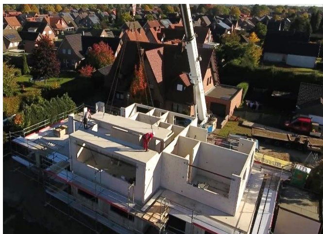
Figure 2 First residential building with load-bearing and non-load-bearing interior walls where the aggregate was replaced by 100% recycled aggregate type 3 (abZ/aBG), Picture: Fa. Büscher, Heek
