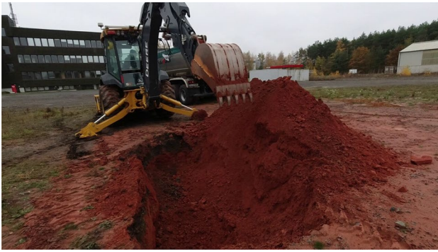
Fig. 8 Final excavated trench
