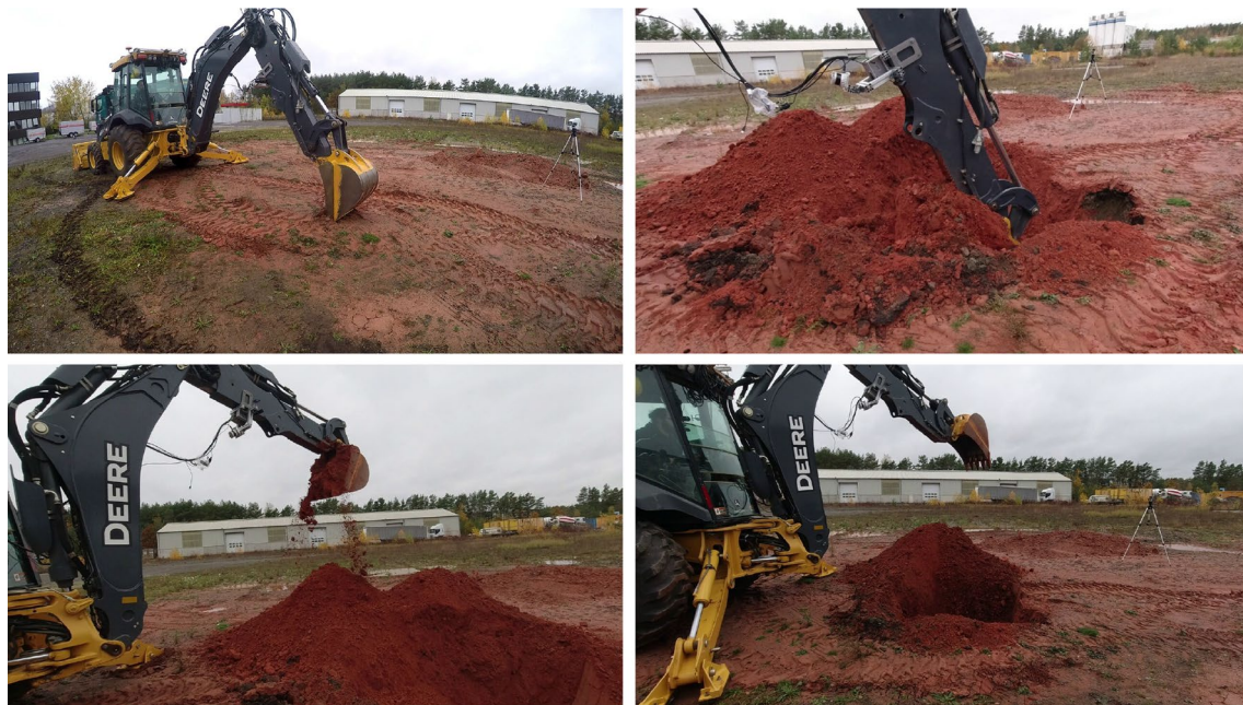
Fig. 5 Image of the start of the four different digging phases of the excavation process. “Digging” (top left), “Move to Dumping” (top right), “Dumping” (bottom left), “Move to Digging” (bottom right)
