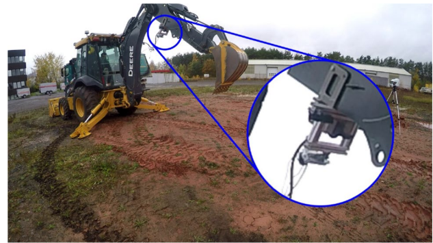
Fig. 2 Backhoe loader with additional sensor system
