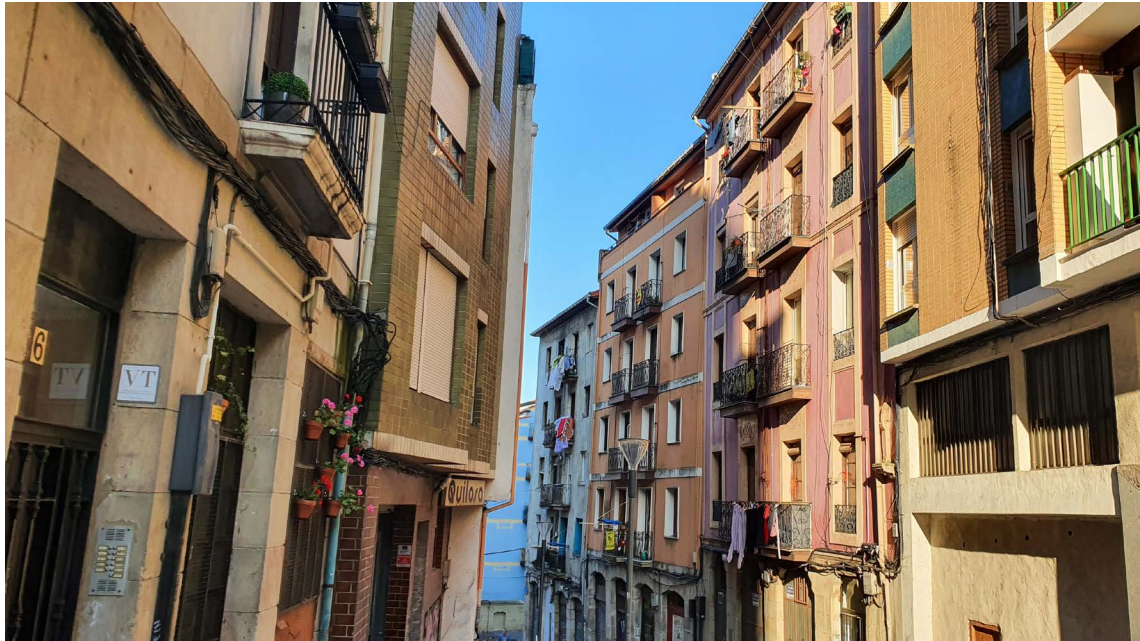
Photo 18: Non-renovated residential buildings in the steep streets of Bilbao La Vieja
