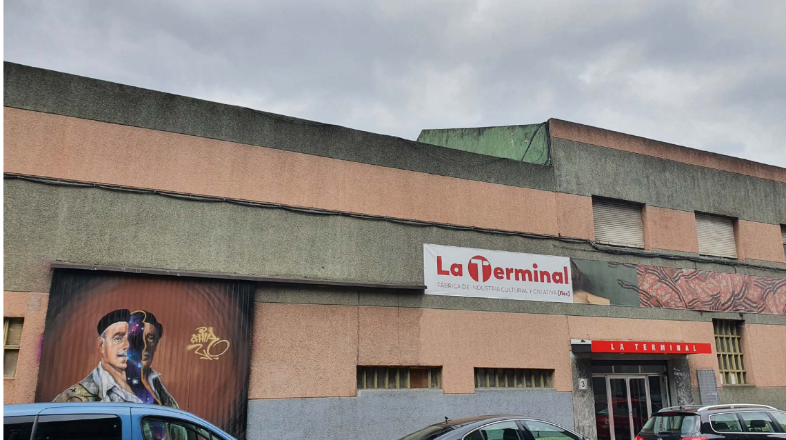
Photo 13: A cultural centre located in an old industrial building as part of the overall strategy of developing an innovation cluster on the island. Source: Author's archive, July 2021
