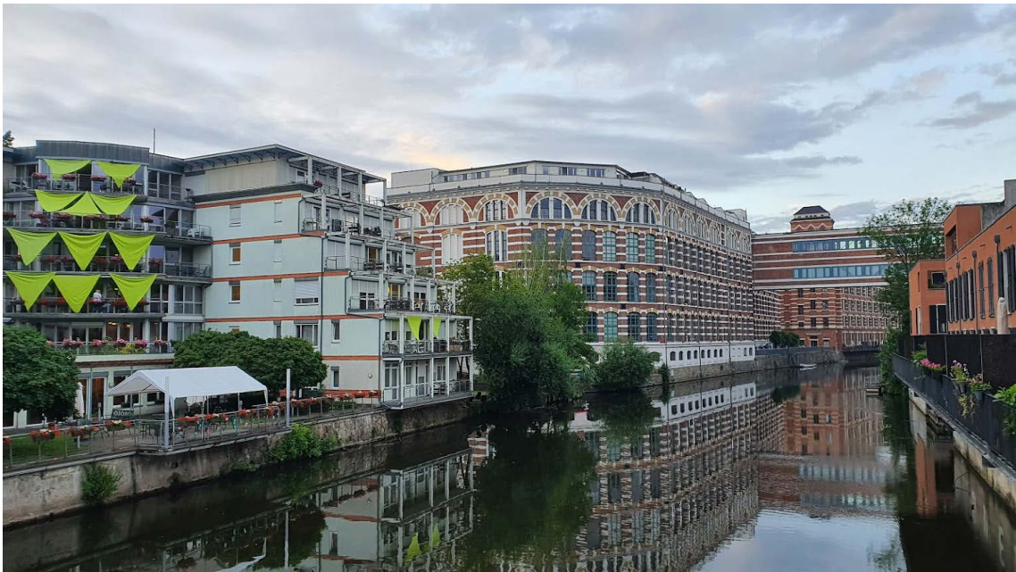
Photo 41: The area along the Carl Heine Canal and the White Elster riverbed where a home for the elderly is constructed close to the business area. Source: Author's archive, June 2021
