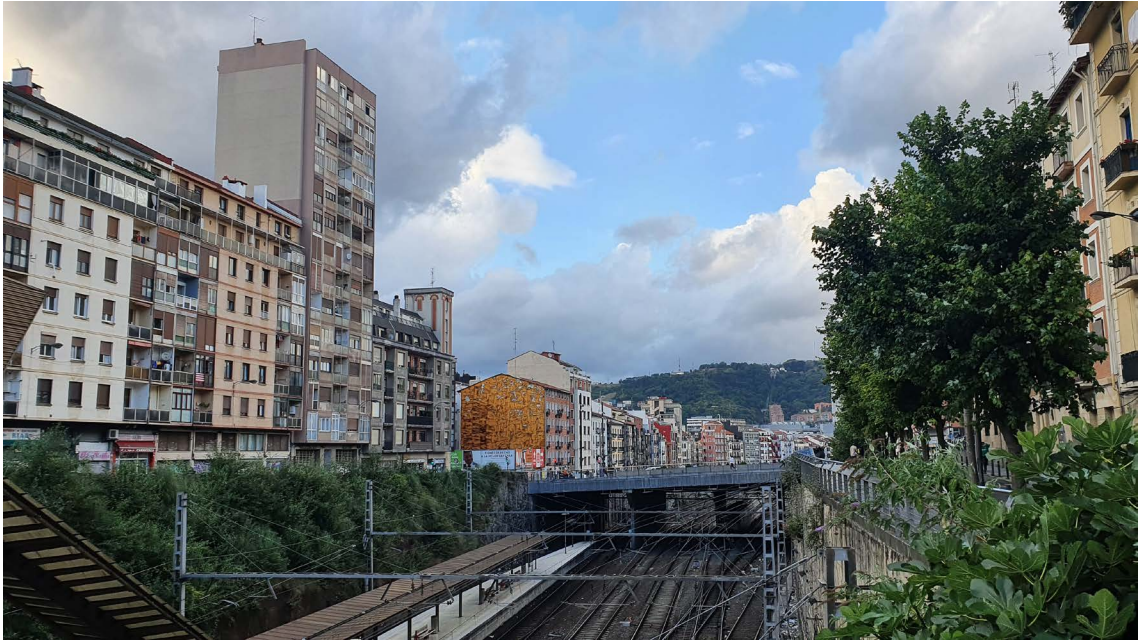
Photo 10: The Zabalburu station and railway trench separating the Zabala neighbourhood (left) and the Bilbao La Vieja neighbourhood (right). Source: Author's archive, July 2021
