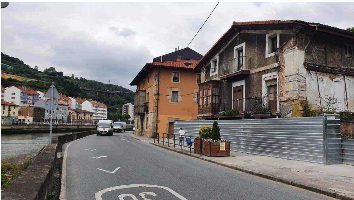
Photo 12: Renovated house (back) and a house set for demolition (front) at Ribera de Deusto street. Source: Author's archive, July 2021
